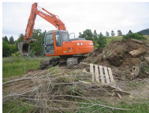
Above: Crook County employee, Morgan Ellsbury, removing debris from dumpsite
