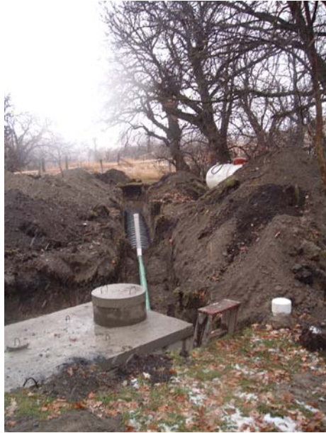
Above: Septic system replacement project using infiltrators for leach field
