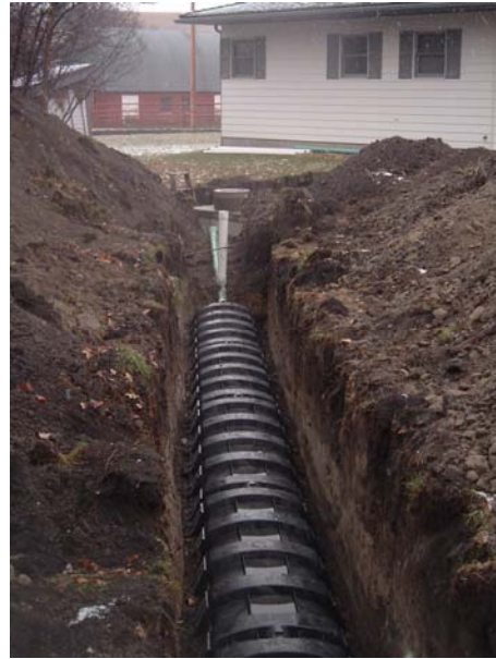
Above: Septic system replacement project using infiltrators for leach field
